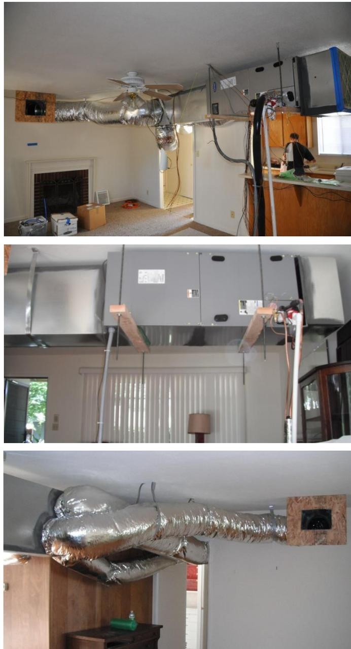
FIGURE 6. TYPICAL REFERENCE HEAT PUMP SYSTEM INSTALLATION WITHIN CONDITIONED SPACE
