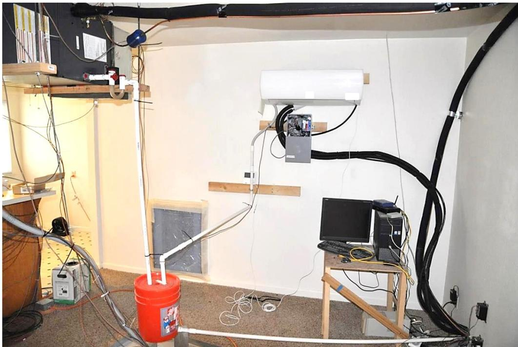
FIGURE 9. WALL-MOUNTED VCHP FAN COIL AND REFERENCE SYSTEM AIR HANDLER AT GRANGE HOUSE
