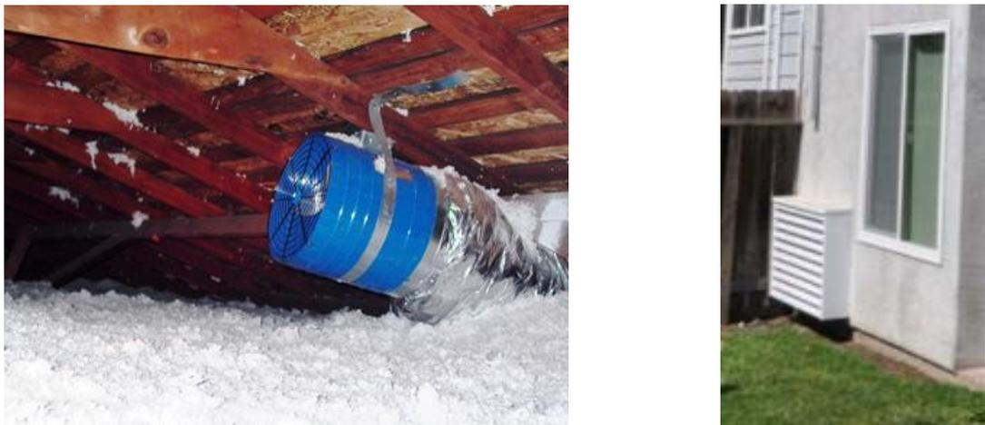
FIGURE 12. WHOLE-HOUSE FAN IN ATTIC AND SIDEWALL OUTSIDE AIR INLET AUTOMATIC DAMPER AT CALEB
