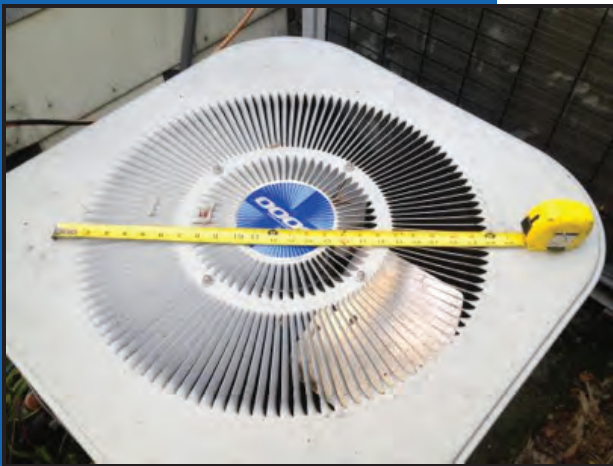
Figure 1- MEASURING THE DIAMETER OF THE CONDENSER
