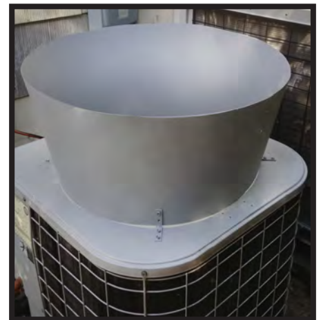
Figure 10- ATTACHING THE DIFFUSER
