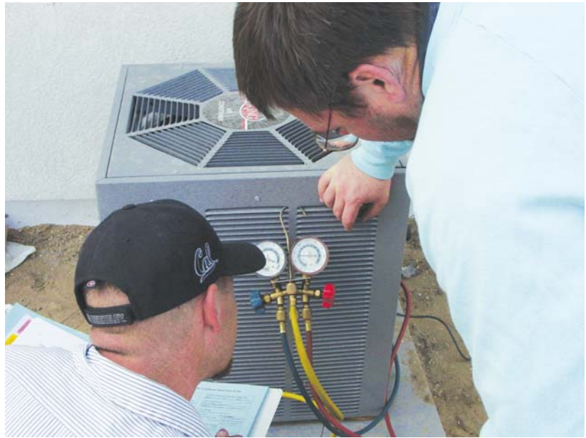
Proper installation takes time and competent technicians.
