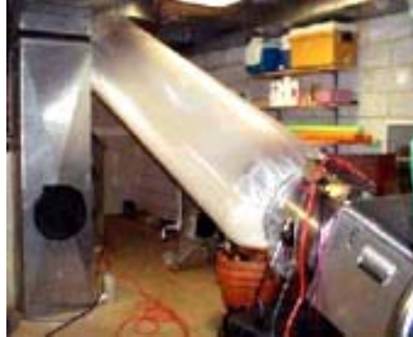
Figure 4.3.9. Carrier/Aeroseal Duct Sealing
