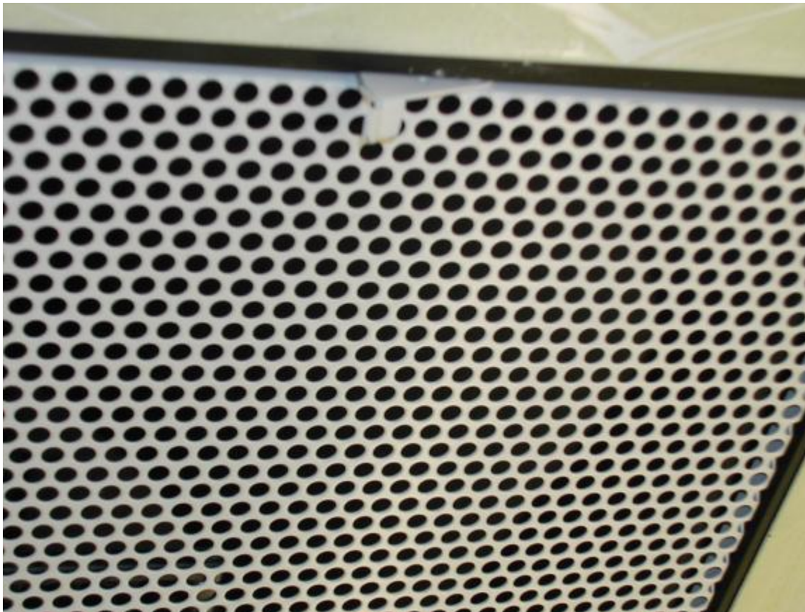
Figure B.1: Clamp on a hinged perforated-plate diffuser. Technicians should always look for clamps and hinges, as the use of foam plugs is always preferable to other diffuser sealing techniques for aerosol injection.
