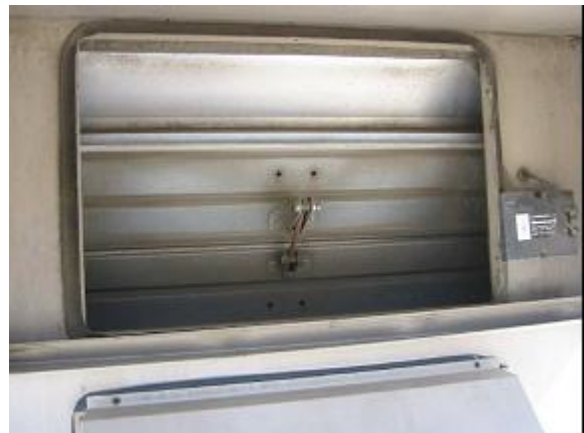
Figure 2.8.2: Damper and sensor module
