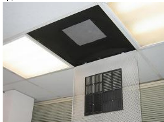
Figure 2.2.2: Foam plug in the central discharge of a hinged diffuser.
