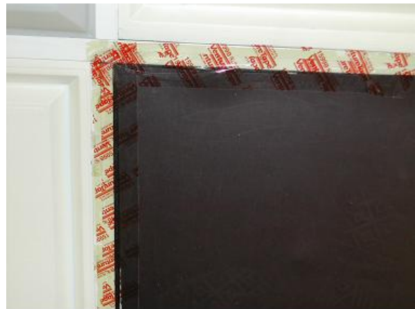
Figure 2.2.1: Plastic film tape above and below a magnetic sheet - diffuser prepared for sealing.
