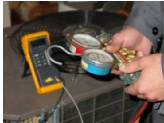
Figure 2.4.4: Measuring refrigerant pressures
