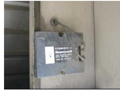
Figure 2.8.4: Enthalpy sensor
