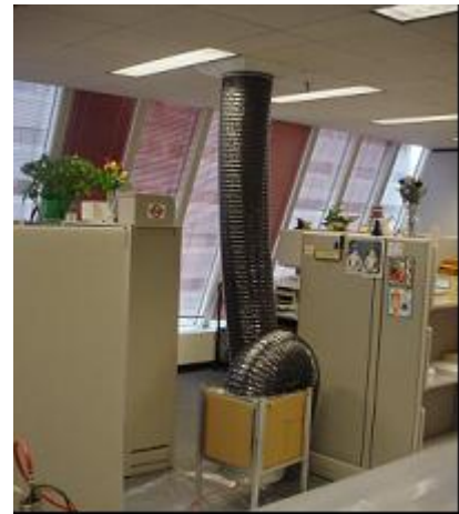
Figure 2.3.2: High-flow scrubber-fan system depressurizes and scrubs particles from a drop ceiling
