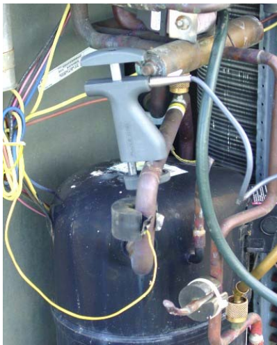
Figure 2.4.3: Measuring suction line temperature with a clamp on thermocouple
