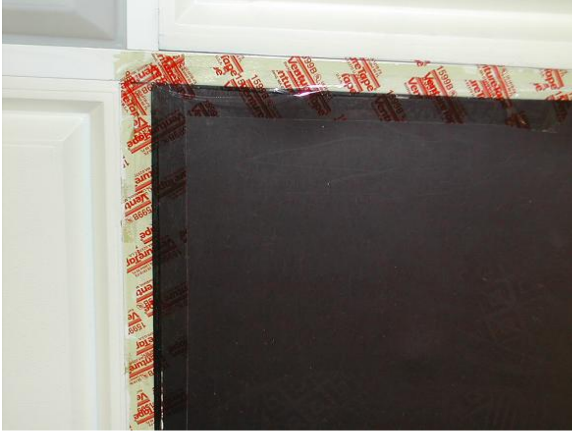
Figure B.4: Plastic film tape installed prior to application of a magnetic sheet to a ferrous perforated-plate diffuser.
