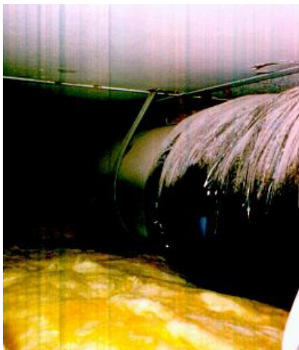
Figure 1.1.2: Drugstore ductwork installed above insulated ceiling tiles
