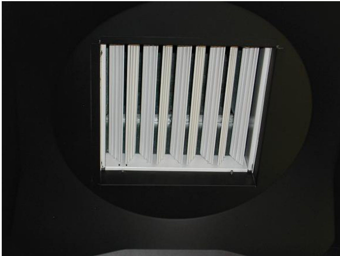
Figure B.2: Recessed internal vanes within a hinged diffuser. When such vanes are not recessed, they can often be removed temporarily.
