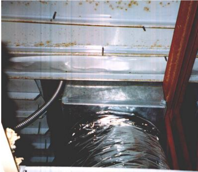
Figure 1.1.4: Uninsulated roof-deck
