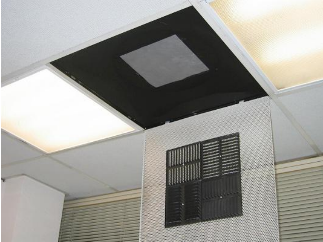
Figure B.3: Foam plug applied to the central discharge, below the recessed vanes of a hinged diffuser.
