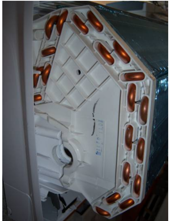
Figure 62 US Model Mini Split Evaporator Coil
