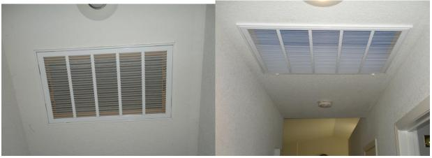
This change lowered the return static pressure from 0.69 IWC to 0.22 IWC and increased the airflow by 19 percent from 289 CFM per ton to 343 CFM per ton. The fan watts dropped from 620 to 350watts.
