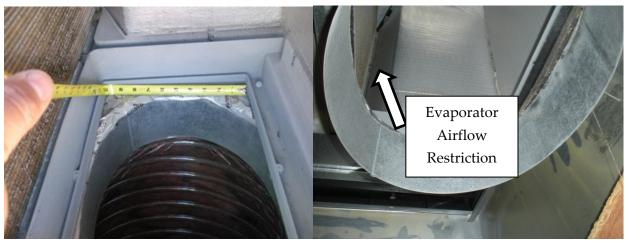
The system has no cooling inlet for the compressor and has melted the insulation on the TXV bulb (Figure 38 and Figure 39).
