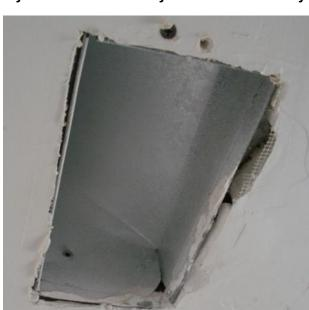
Figure 48: System 74—One of Many Boot and Boot-to-Drywall Leaks
