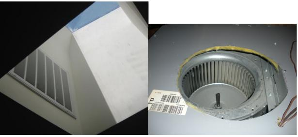
This change resulted in lowered the return static pressure from 0.69 IWC to 0.16 IWC and increased flow from 253 CFM per ton to 386 CFM per ton. The Sensible Efficiency was improved by 18.5 percent.
