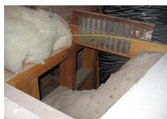
Figure 57: Leakage between Conditioned Space and Attic
