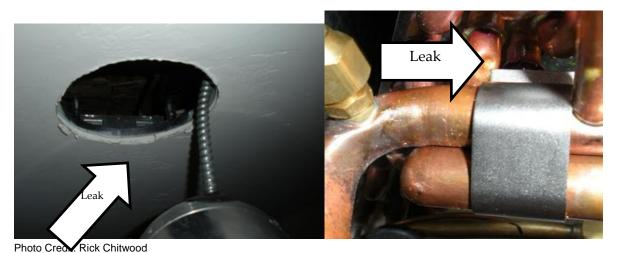
Figure 46: System 74—Refrigerant Leaks
