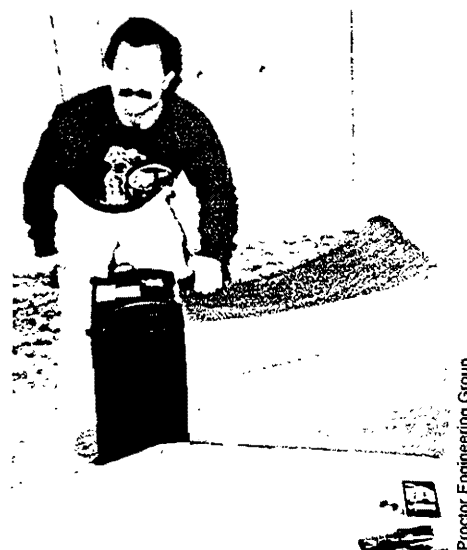
An air conditioning technician with the Auburn Heat Pump Project uses a flow hood, a diagnostic tool used to measure the amount of air flowing through the open grille of a duct system.
