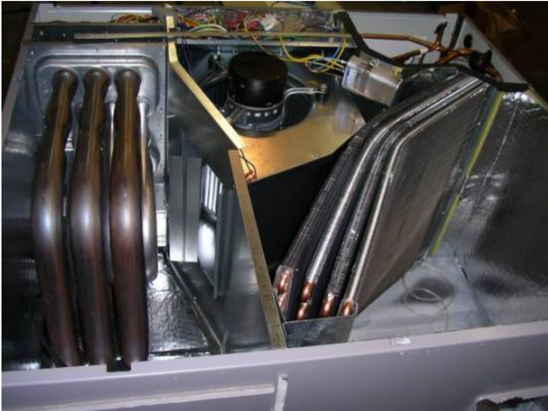
Figure 32: Package Unit Initial Indoor Section Configuration
